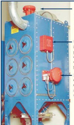
Explosion Suppression Cannon™ mounted at Dust Collector inlet prevents flames from expanding upstream.
